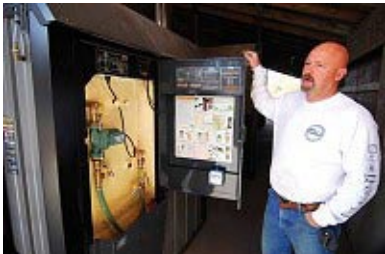
a holding tank that uses wood to heat 400 gallons of water as part of a system that provides heat and hot water to Pierce's home on Friday afternoon in Arriola.
